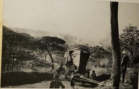
Hauling boats up steep incline by block and tackle.
